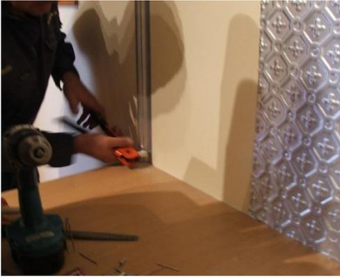
If a Pressed Metal Border is also being used this can be put into place now as the panels will sit inside or underneath this. This is done using Liquid Nails and a nail or rivet.
